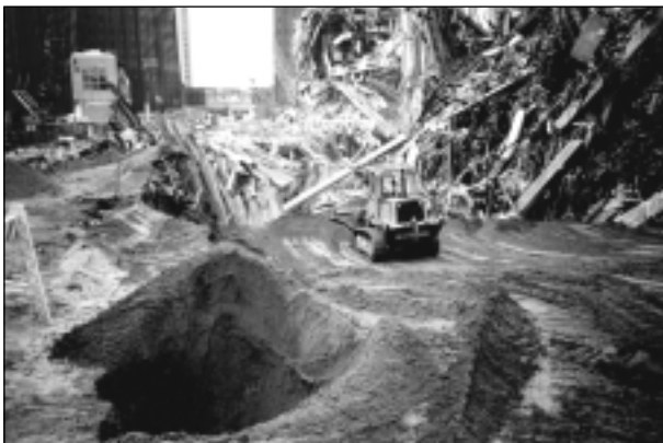
FIGURE 8 Backfill operations at Liberty Street.
