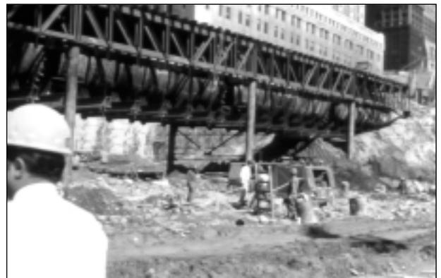
FIGURE 4 Original PATH tube suspension system.
