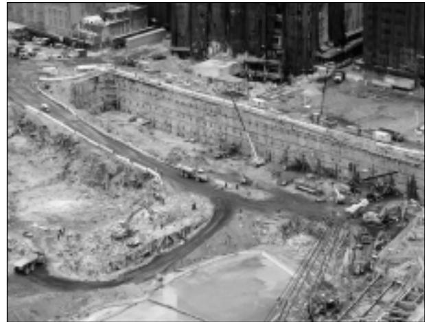
FIGURE 11 Progress along the Liberty Street slurry wall showing the installation of the fourth-tier anchors.
