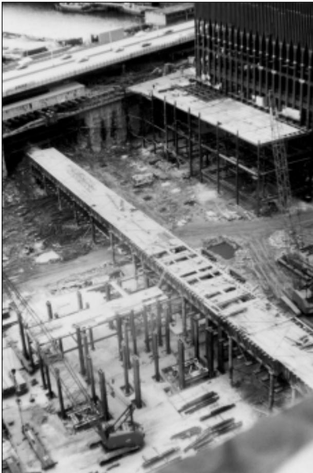
FIGURE 5 Original excavation, WTC 1 steel core started, PATH tubes temporarily supported while new station is constructed along Greenwich Street slurry wall.
